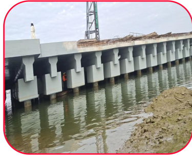
码头涂层防腐
